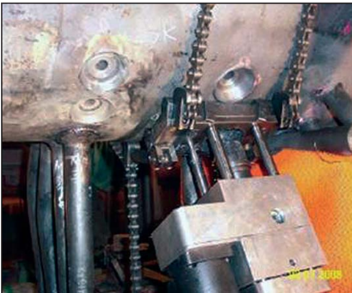
Boiler Tube Stub Drilling
