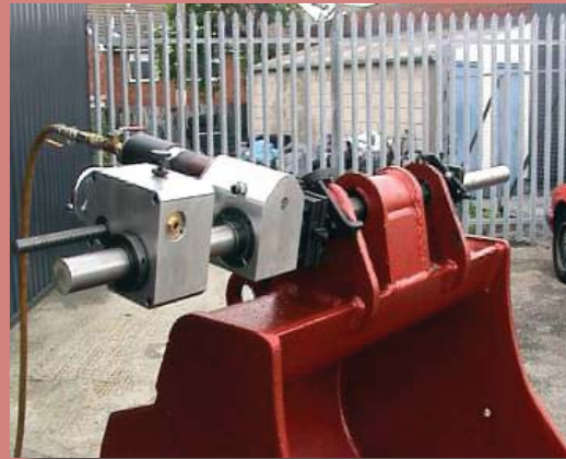
Bucket Line Boring and Repair
