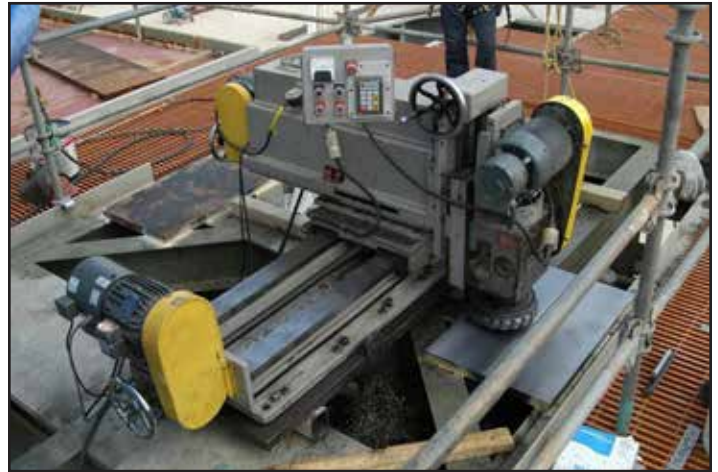
In-place Machining with Mactech's Master Mill
