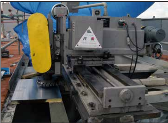
On-site Motor Base Milling
