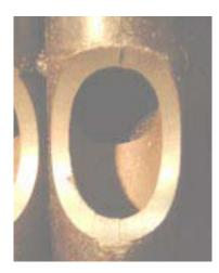
Over time waterwall tubes corrode on the inside, resulting in the need to replace or repair them. Typically only one side of the tube is accessible for repair. Current practices include torch cutting the damaged section, hand grinding and rewelding the hole. This process is time intensive and the holes are typically inconsistent in size and shape. This causes welding to be difficult and the need to fabricate individual caps.
