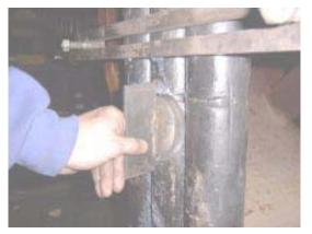
We can machine coupon windows in virtually any location on a water wall tube, whether it is ten in a row or ten individual cuts. The process is much more efficient than conventional methods, results in consistent hole size, and the caps enable efficient weld up of the hole. Currently coupon windows can be cut in 1.5" to 3" diameter tubes.
